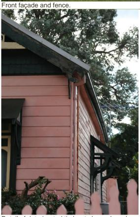
Detail of deteriorated timber to barge board.
